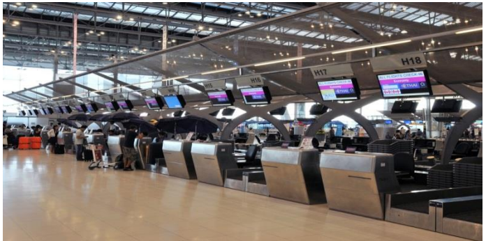
Airport Display Systems
