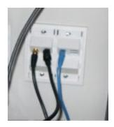
MuxLab products may be applied to this approach by installing the appropriate MuxLab balun behind the wall outlet using multimedia feed-thru couplers. Feed-thru couplers pass the audio-video cable connector through the outlet so that they may be accessed behind the wall. In order to support Cat5, an audio-video balun must be connected behind the wall. The result is an aesthetically pleasing installation that supports Cat5 behind the wall.
